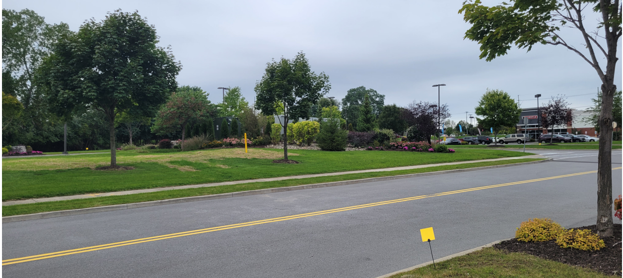
Walmart Plaza charging station transformer and landscaping, photo by submitted by Aaron Sweeney, September 21, 2022.
