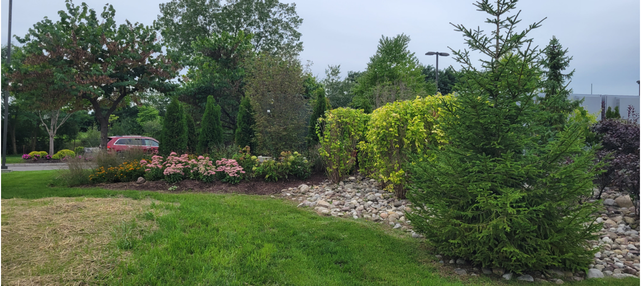
Walmart Plaza charging station transformer and landscaping, photo by submitted by Aaron Sweeney, September 21, 2022.
