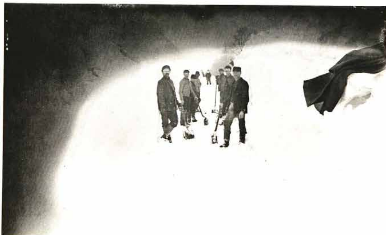
TUNNEL OF SNOW - SOUTH OF FRIENDS MEETING HOUSE NOW COUNTY ROAD 8 CHARLES H. GARDNER, MYRON COTTON
